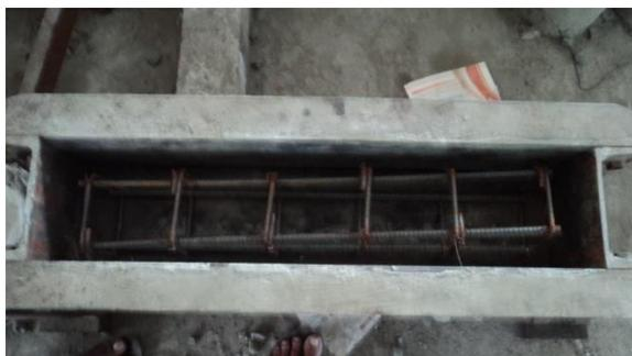
Figure 6. Reinforcement cage in the mould
