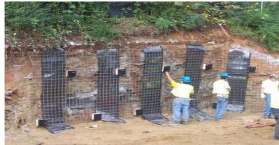
Figure 4: Soil Nailing
