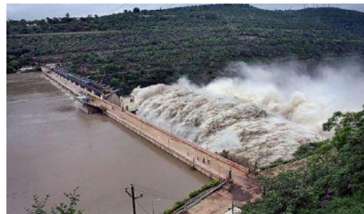
Figure 2 and 3. Srisaillam Dam Had Tilted But Regained Its Position
