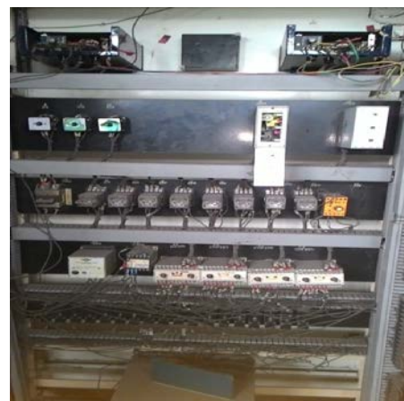
Fig. 3 Relay Control Logic of SWCS
