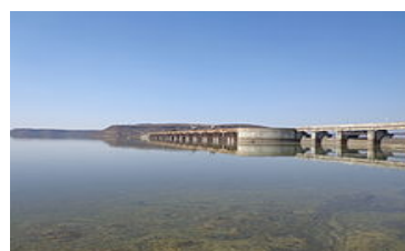
Fig.1 Tighra Dam Located Near Gwalior
